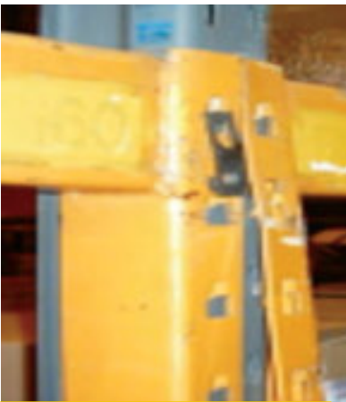
Disengaged beam end plate
