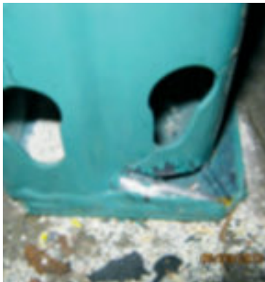
Torn footplate weld
