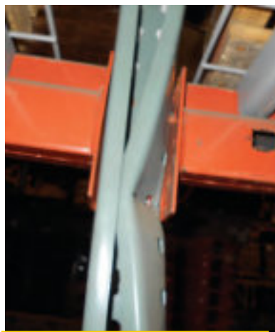
Damage behind beam connector
