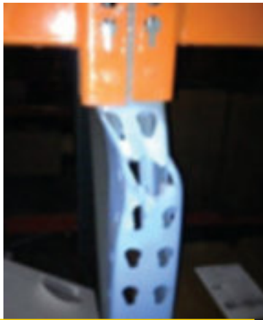
Damage under beam level
