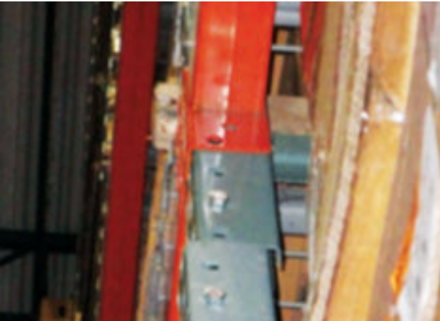
Improper splice installation
