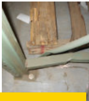
Roll formed horizontal strut damage
