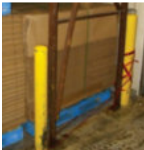
Missing horizontal struts
