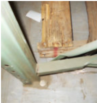
Broken strut connection
