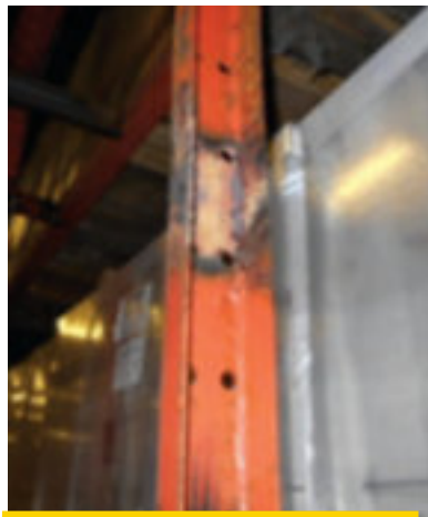
Structural column damage
