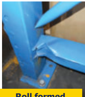
Roll formed closed tube horizontal strut damage
