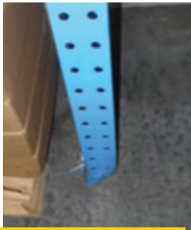
Structural column damage
